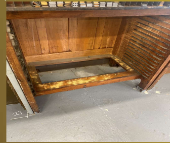
Borer infestation in a type cabinet
