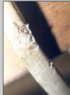
Holes for wires and pipes, mouse staining on corrugated plastic pipes, and a chewed electrical cord
