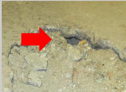
Examples of holes in foundations
