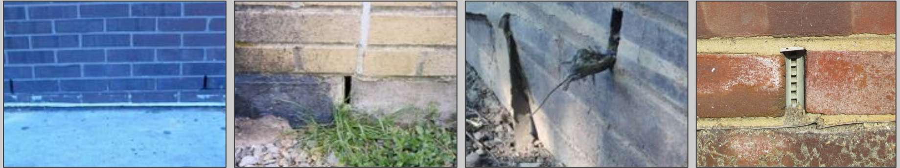
Examples of weep holes: first 3 images are open and the last is closed with an exclusion cover
