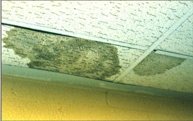
Evidence of mice in the office: urine staining on ceiling tiles, food waste hoarded in an office, and a mouse chewed food container
