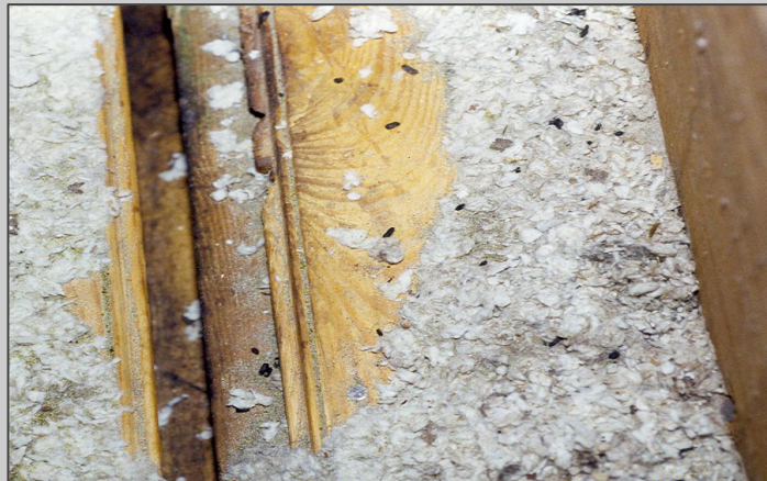
Evidence of mice in the attic around cable chases, floorboards, and pipes
