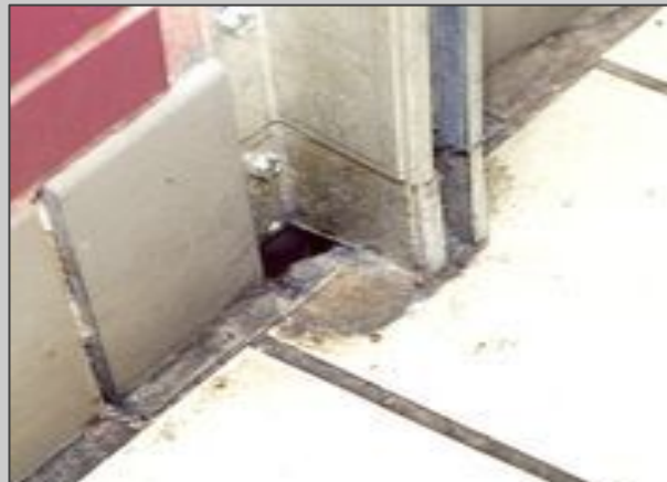
Examples of gaps under garage doors and a schematic for closing the gap
