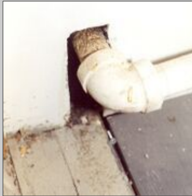
Examples of vent and pipe holes/gaps
