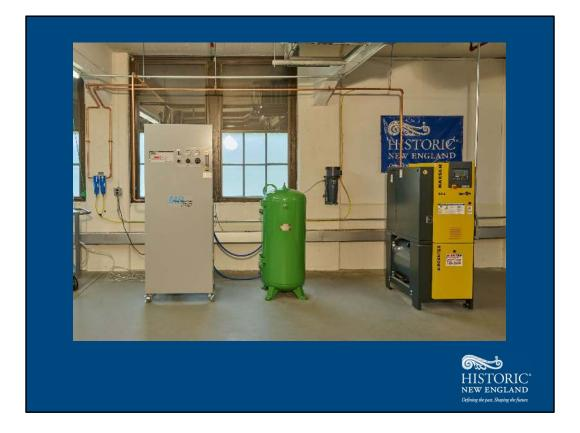
By last year at this time the air compressor and nitrogen generator had arrived. The compressor on the far right is a rotary screw air compressor made by Kaeser and the nitrogen generator on the left with buffer tank in the middle is a Parker Pressure swing Adsorption (PSA) generator that can reach 99.99% nitrogen purity. Here is a picture of it fully installed with electrical and plumbing.
