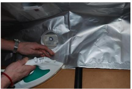
Remember to pad out sharp corners that might pierce the film. As with the custom chambers, begin to seal the edges, leaving room for the vacuum nozzle. Vacuum out as much oxygen as possible
