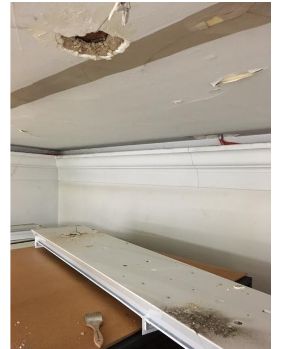
Building 8, 4th floor mezzanine, showing removed light fixture and phone line leading into the ceiling
